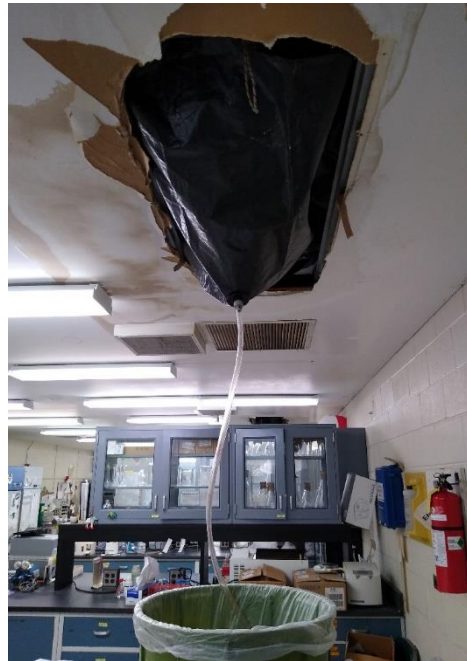
Roof membrane leak impacted lab below
